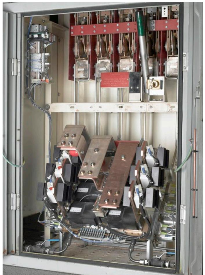
You retain your existing cubicle, overhead bus-work, and cabinet doors. We replace the diode rectifier, replace the on-line repair switch, replace the manifolds with stainless piping
