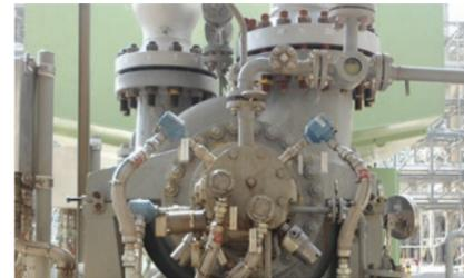
Increased vibration levels were detected on a boiler feed pump being returned to service at the end of a major planned outage. The Bently Nevada condition monitoring system enabled plant personnel to diagnose and fix the problem without delaying the startup schedule and declaration of full plant availability. \$90,000 USD in contract penalties were avoided, as well as potential damage to the machine.
