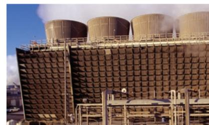
A plant lost more than \$300,000 USD to cooling tower fan problems before installing permanent monitoring. In one instance, a blade sheared off completely. The resulting unbalance destroyed the entire fan assembly and parts of the tower, even though simple vibration switches were installed and a portable data collector was being used to check the fans monthly. After permanent monitoring systems were installed, no further failures have occurred.
